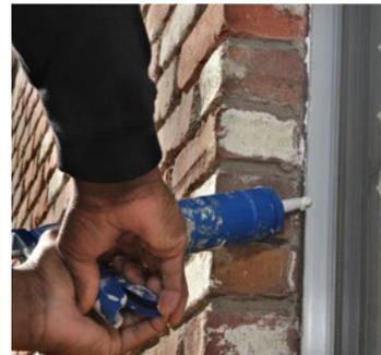
**CAUTION:** When sealing any home, be aware of the dangers of indoor air pollution and combustion appliances referred to as backdrafts. Backdrafts occur when various combustion appliances and exhaust fans compete for air. An exhaust fan may pull the combustion gases back into the living space. This can create a very dangerous and unhealthy situation in the home.
